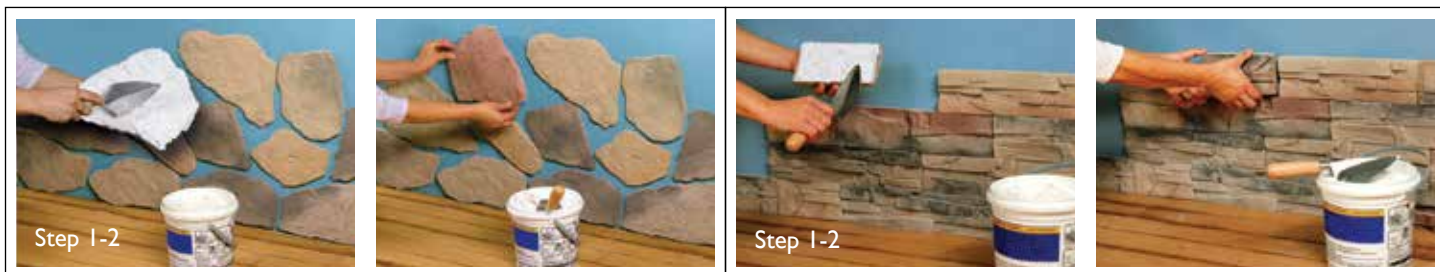
Springbrook, River Stone. Mastic Adhesive and 1/4" joints for grouting.
