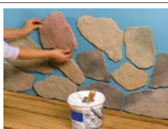
Springbrook, River Stone. Mastic Adhesive and 1/4" joints for grouting.
