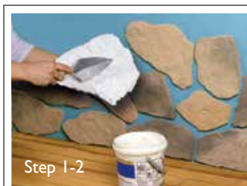
Springbrook, River Stone. Mastic Adhesive and 1/4" joints for grouting.
