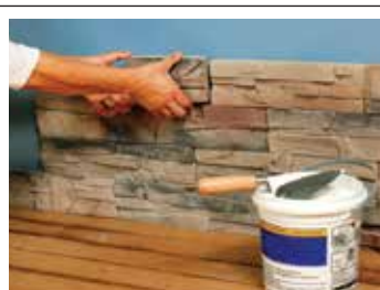
Roma, Rocky Mountain LedgeStone. Mastic Adhesive, stacked tight. NO grouting.
